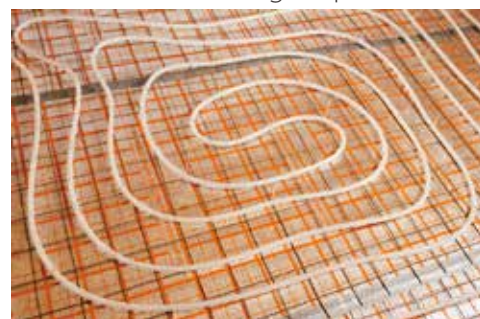
Floor heating loop
